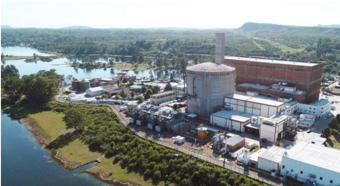
Figure 5. Photo of the Embalse nuclear power plant
