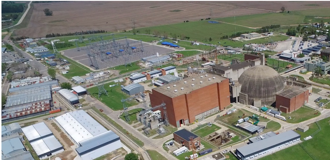
Image 03: ATUCHA II nuclear POWER PLANT
