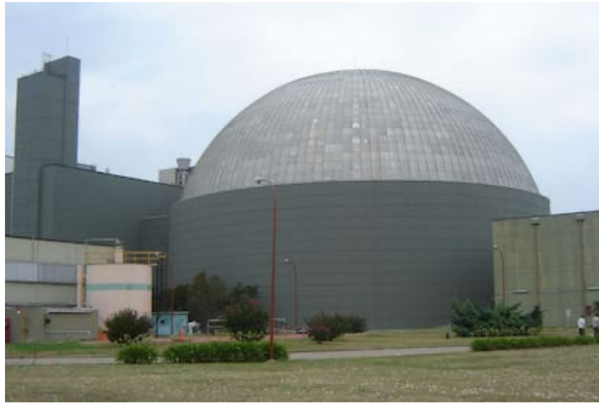
Figure 4. Photo of the Atucha I nuclear power plant
